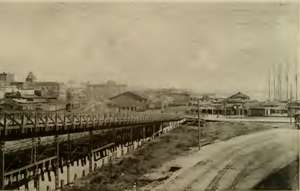
R. R. YARDS FROM THE VIADUCT.
